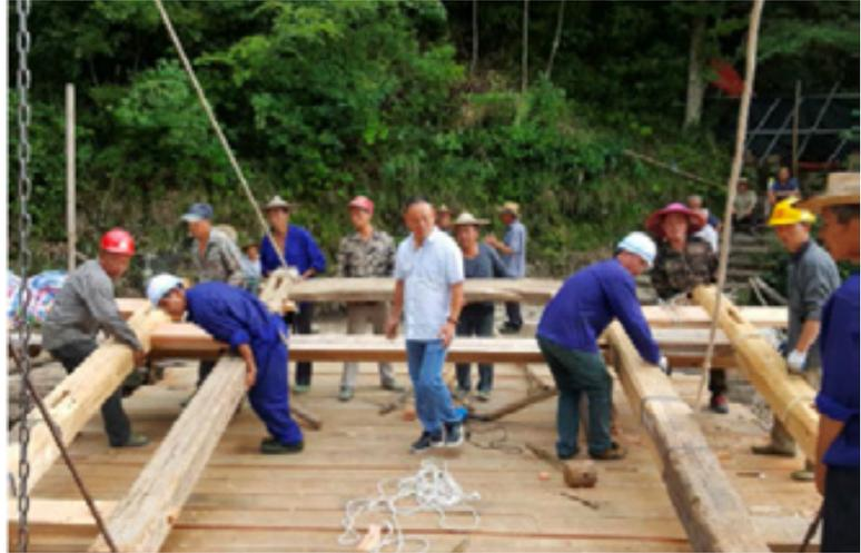
► **Fig. 25.** Cooperation in action: carpenter guides work in reassembling a bridge beam frame, Xuezhai Bridge, Taishun County Wenzhou City, Zhenjiang Province, China (Source: Huang Zi)
