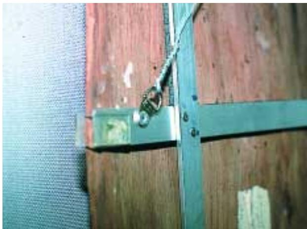
Mount system with D-rings and polycarbonate clips in place.
