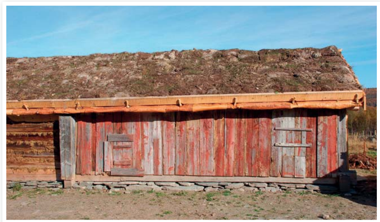
59: Rasmusvollen after repair by the Outbuildings Project
