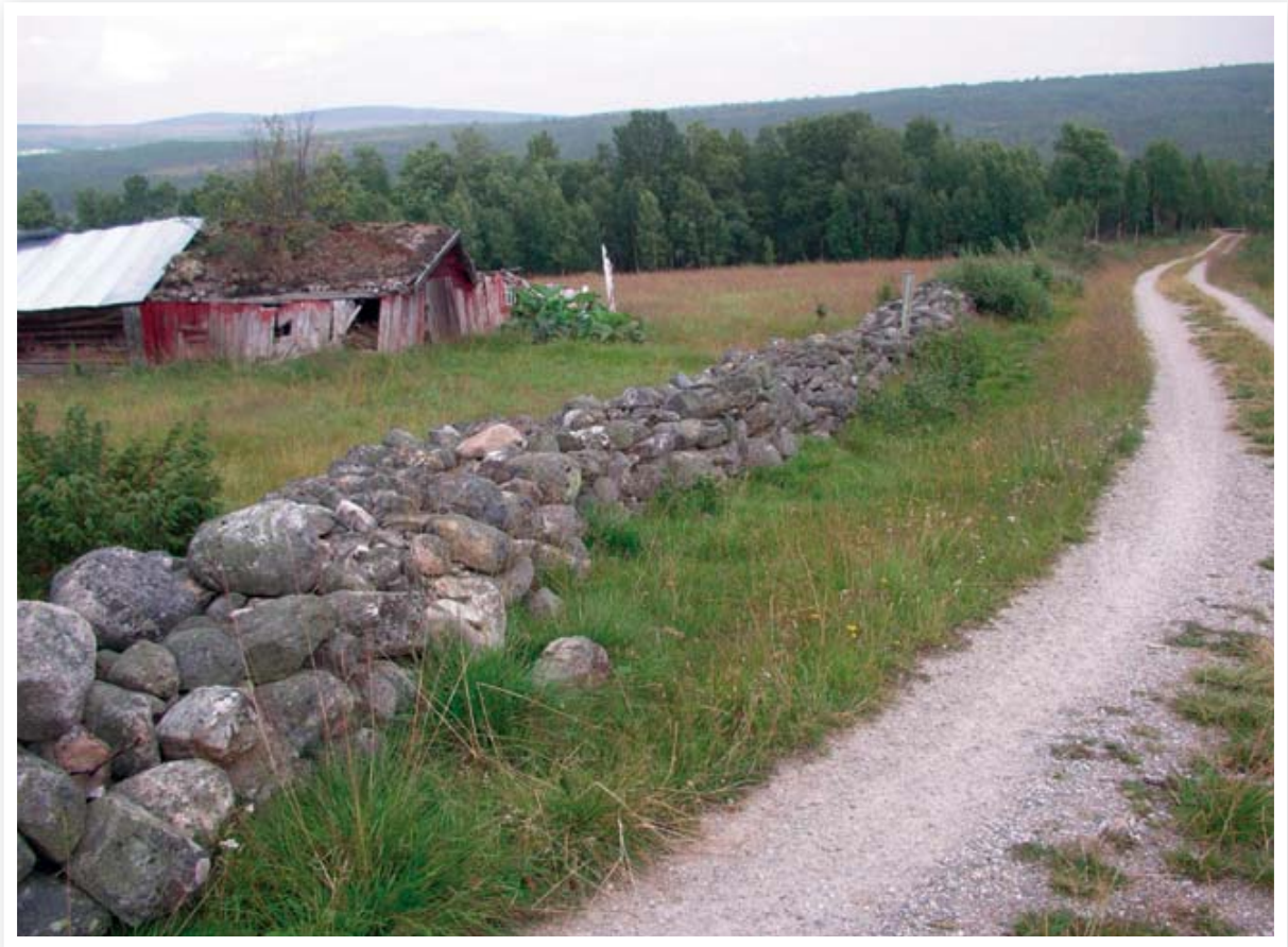
60: Rasmusvollen before repair
