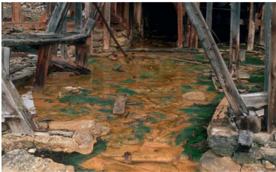
71: Christianus Sextus Mine – polluted ground under the cableway station.
