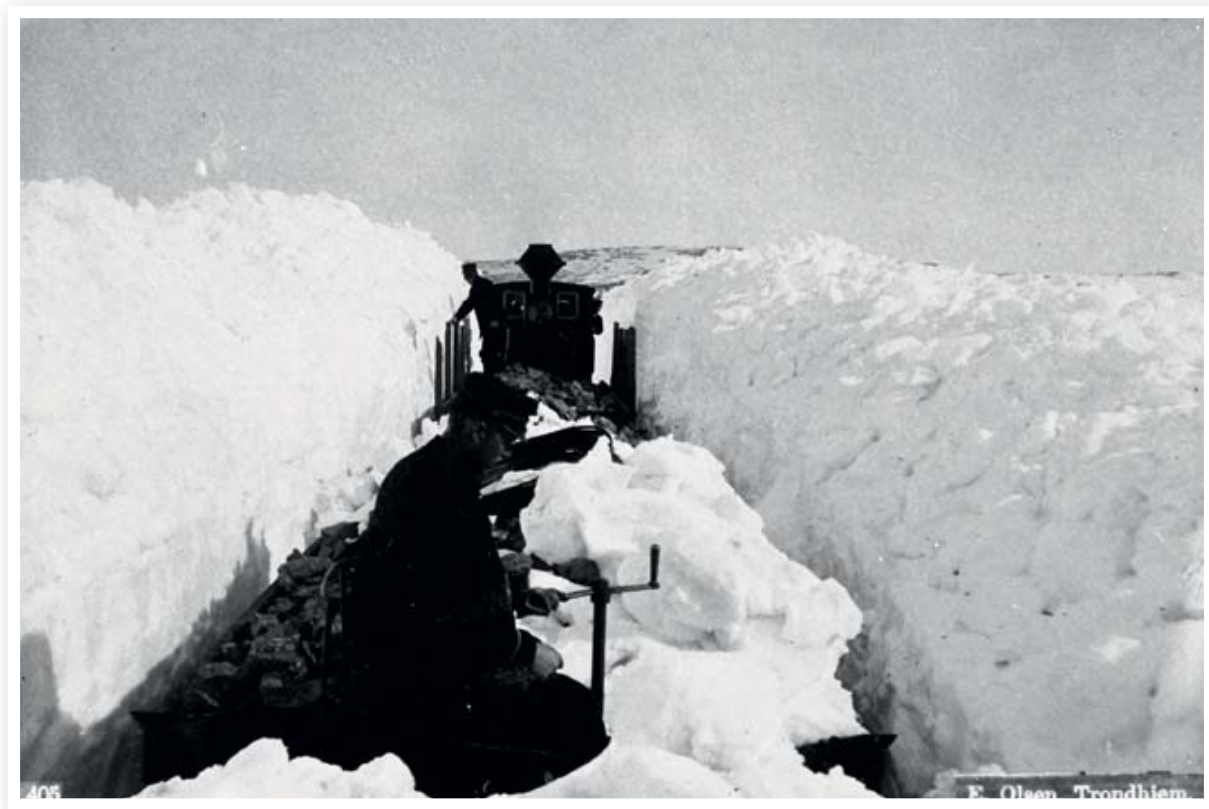
75: Arvedalslina – a sidetrack to the main railroad from Oslo via Røros to Trondheim. The track, established 1886, went up the hill to the King's Mine. It was always difficult to keep open in the winter and in 1910 it was replaced by a cableway.
