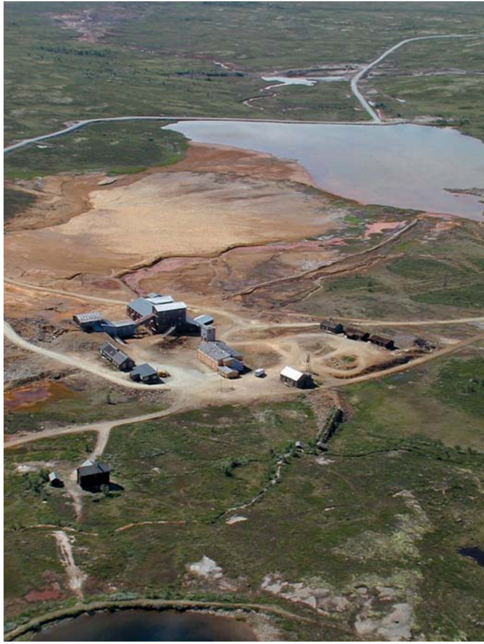
64: Lower Storwartz with the flotation plant.
