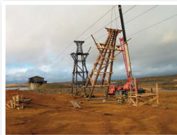
63: Restoration of the cableway – raising a new pylon.
