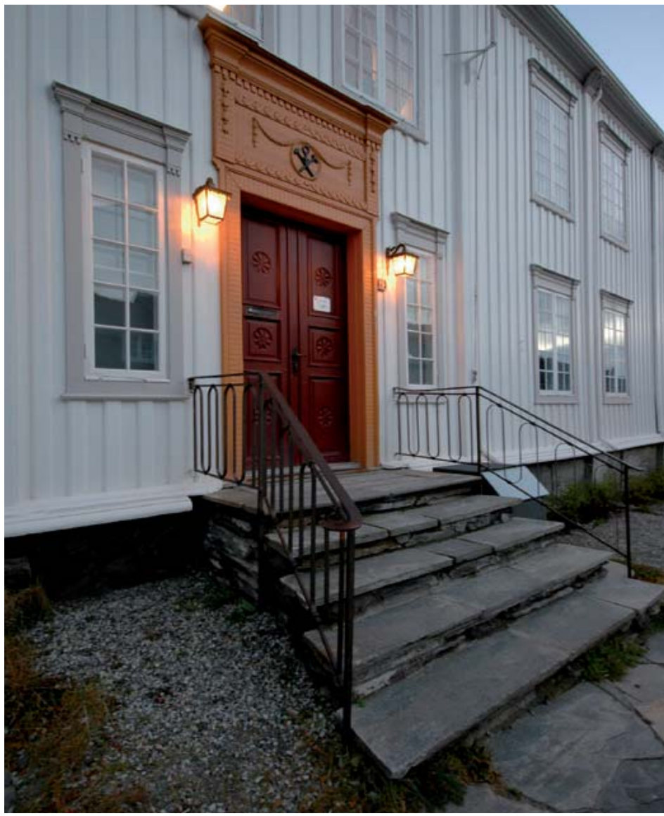
31: Catharina Borchgrevink's house – residence of the bourgeoisie. Presently used as town hall.
