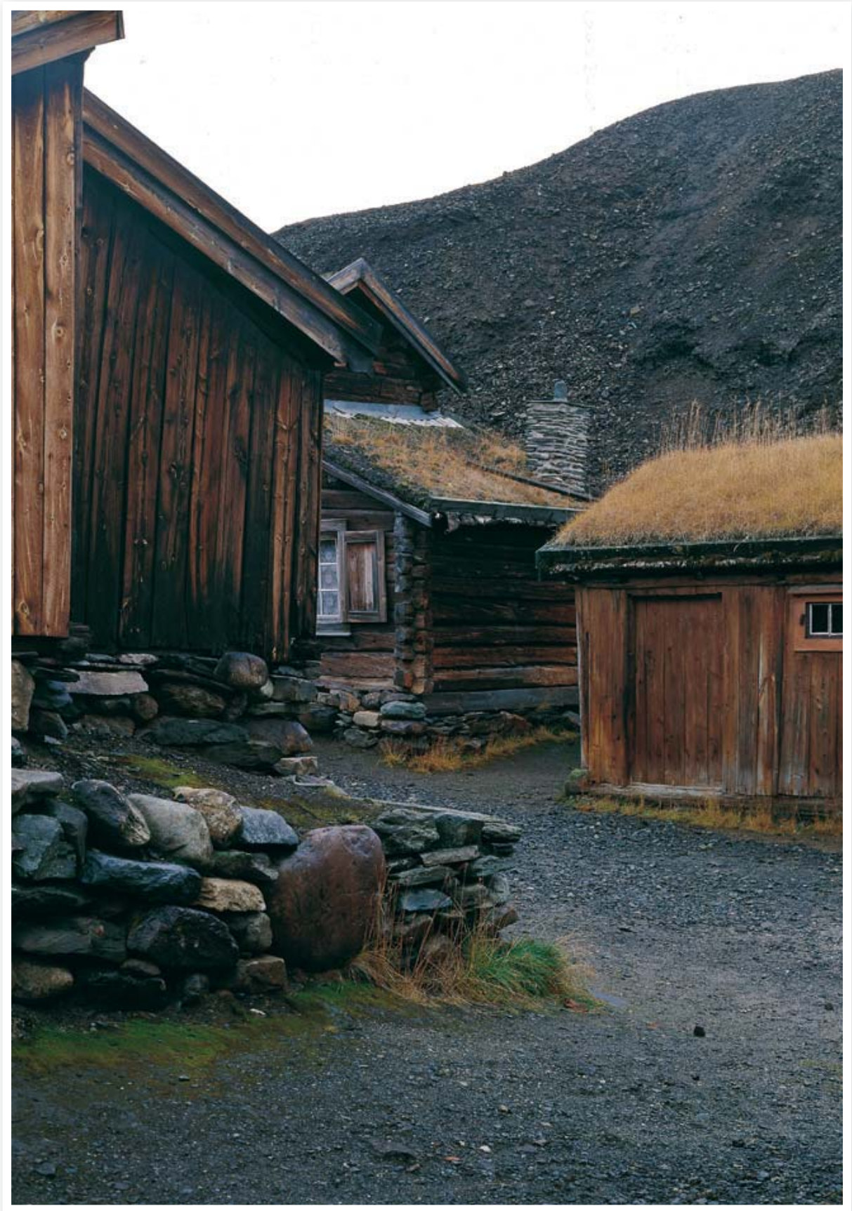
45: The slagheaps with Sleggveien and Tyristuggu in front .
