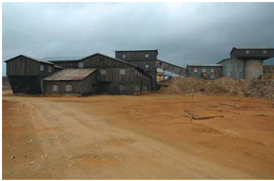
67: The flotation plant at Storwartz.
