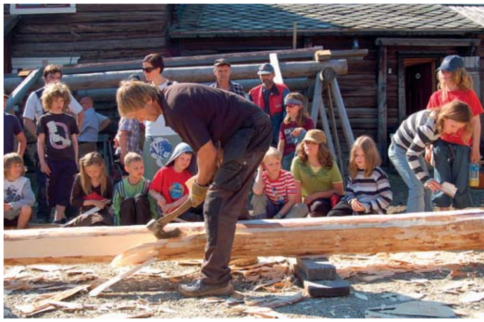
105: Craftsmen at work for the Outbuildings Project.
