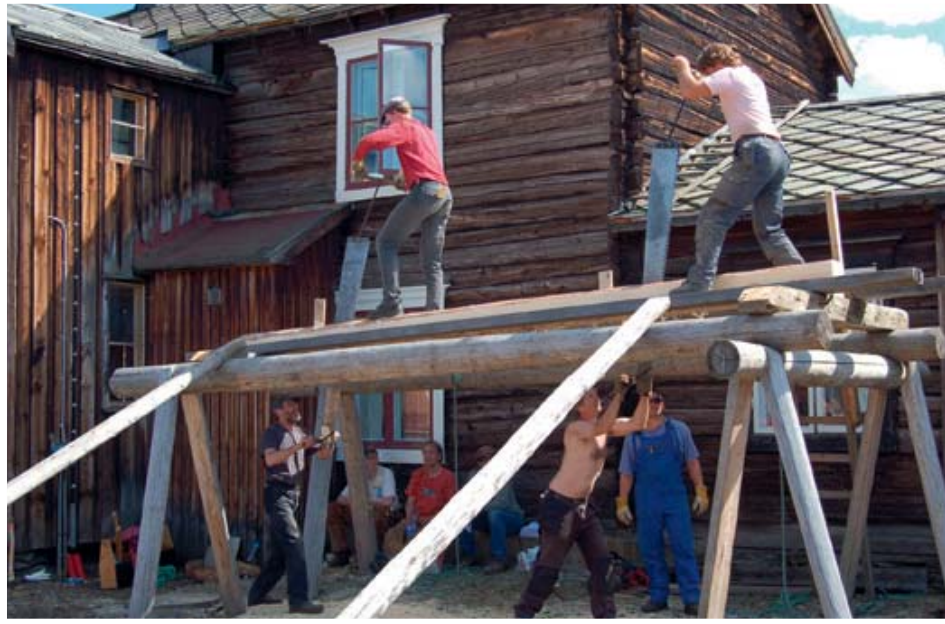
106: Craftsmen at work for the Outbuildings Project.
