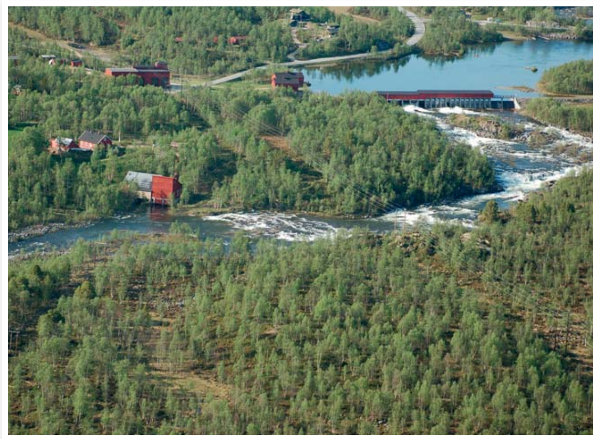
76: Kuråsfossen power station.
